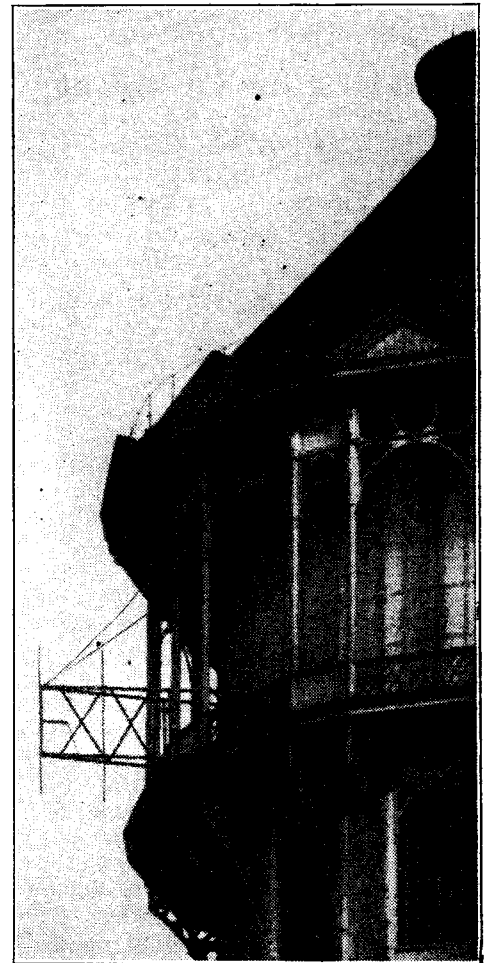
The vision aerial on the south tower of the Crystal Palace. Behind the di-pole aerial is the reflector. A feeder line connects through to the transmitter at ground level.
